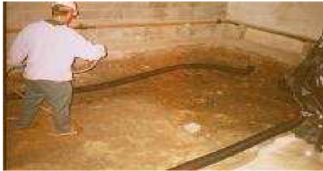
Figure 2. First application of biodispersion product after wetting the soil with municipal water. Black air vent tubes are seen in the background.
