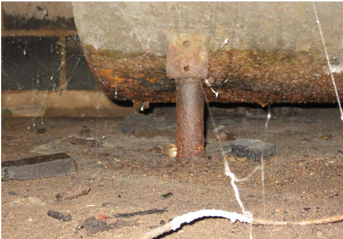
Figure 1. Before application of VaporRemed.
