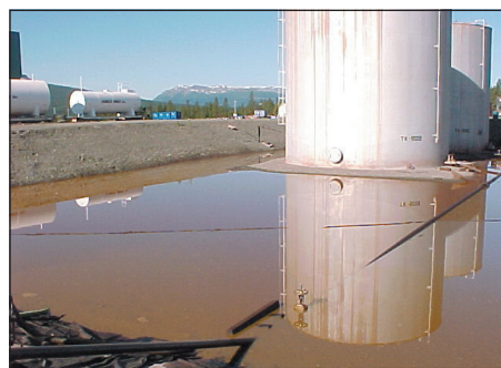
The berm after six weeks' remediation
