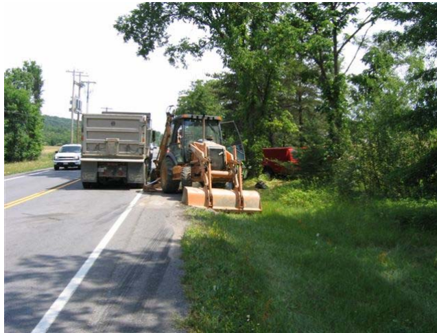
Figure 1. Accident site showing the asphalted road affected by spill.
