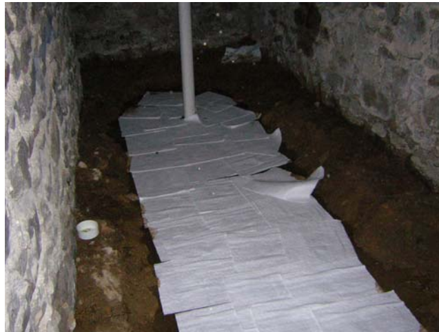
Figure 1. Basement immediately after removal of dirt
