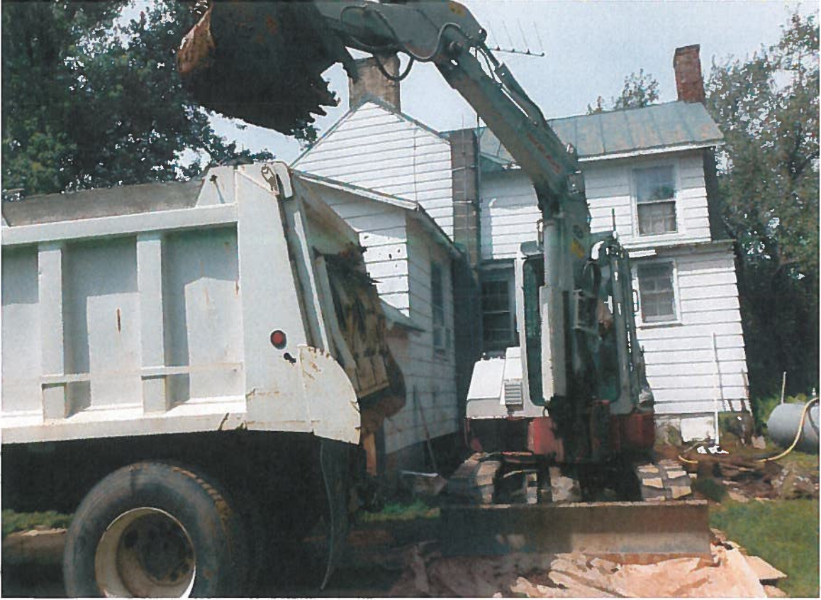
Over-excavation of petroleum-contaminated soils
