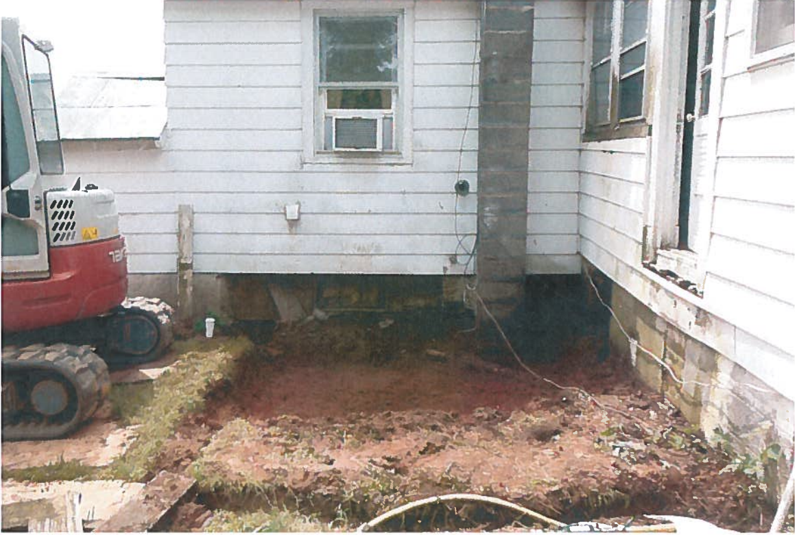
Extent of the over-excavation
