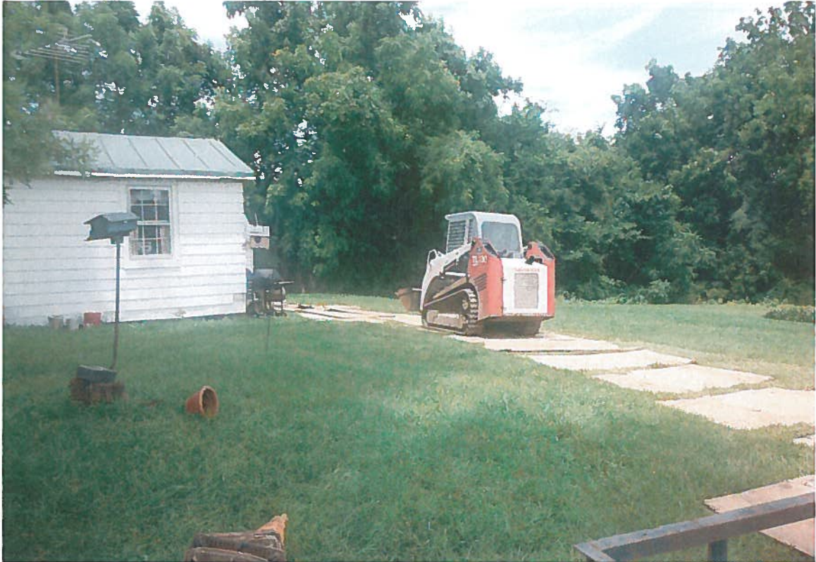
Skid steer loader used for backfilling
