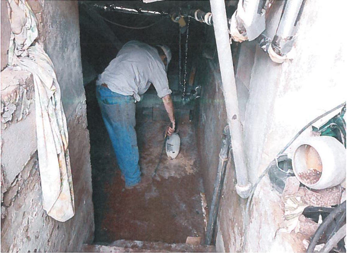
VaporRemed sprayed in the cellar
