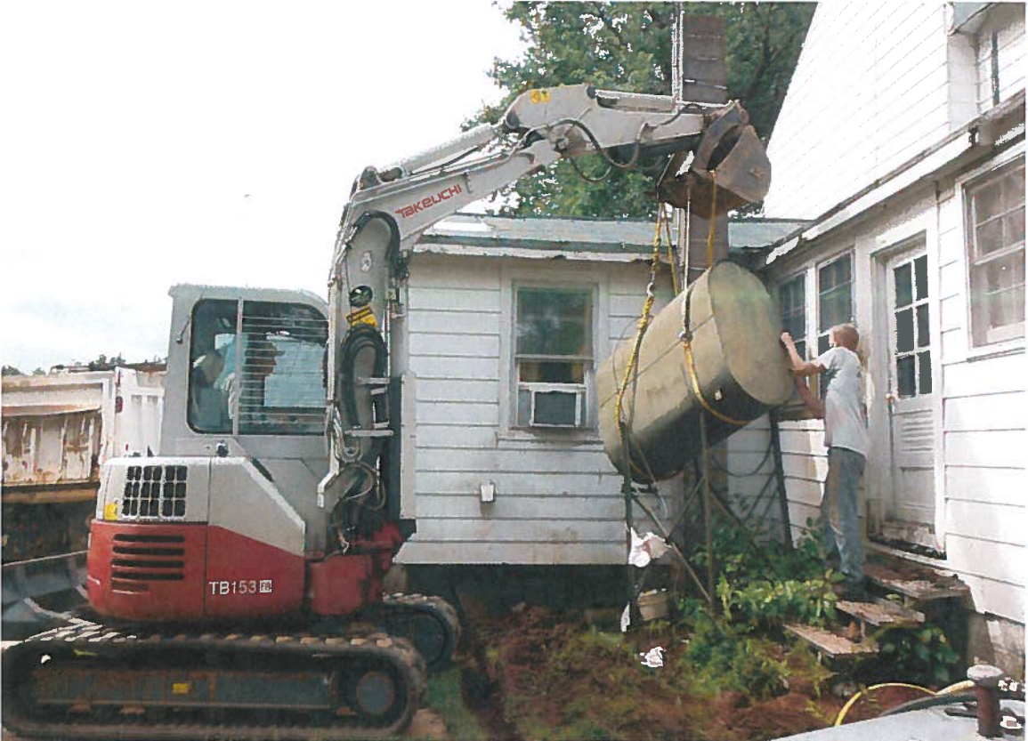
Removal of 275-gallon AST
