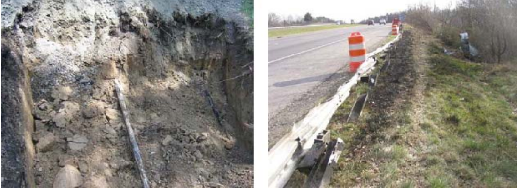
Figure 7 (Left) showing the accident site with the underlying cables on left preventing excavation of soil and Figure 8 (Right) the site of in situ bioremediation.
