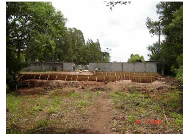
Atuba Project Site: construction of irrigation canals.
