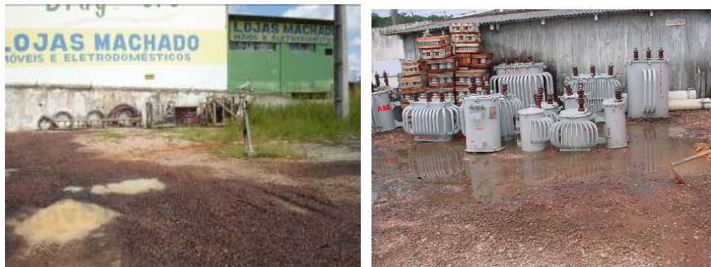
Figure 1 & 2. Mandirituba Power sub Substation and the transformers
