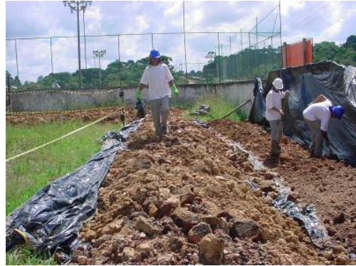
Figures 2 and 3. Excavation of contaminated soil and piled up as stacks.
