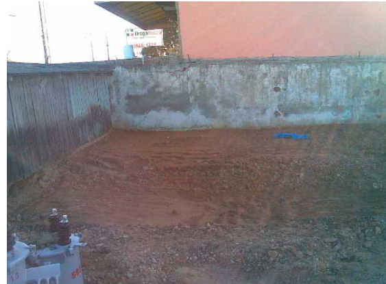
Figure 5. Soil filled back in the pits
