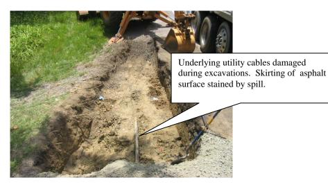
Figure 6. Showing underlying cables and stained skirting of pavement.
