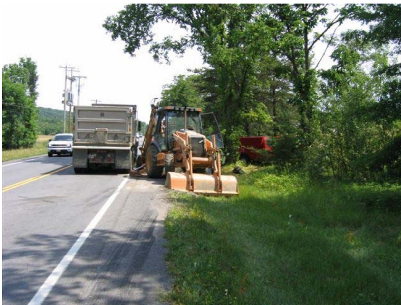
Figure 3. Accident site showing the asphalted road affected by spill.
